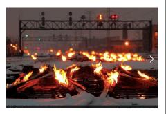
today's heaters are that they can operate over a long time, and many can be started and shut off remotely. Track insulation can be applied to the rails to minimize the heat loss. Rails only need to be warmed to just above freezing to be effective.
